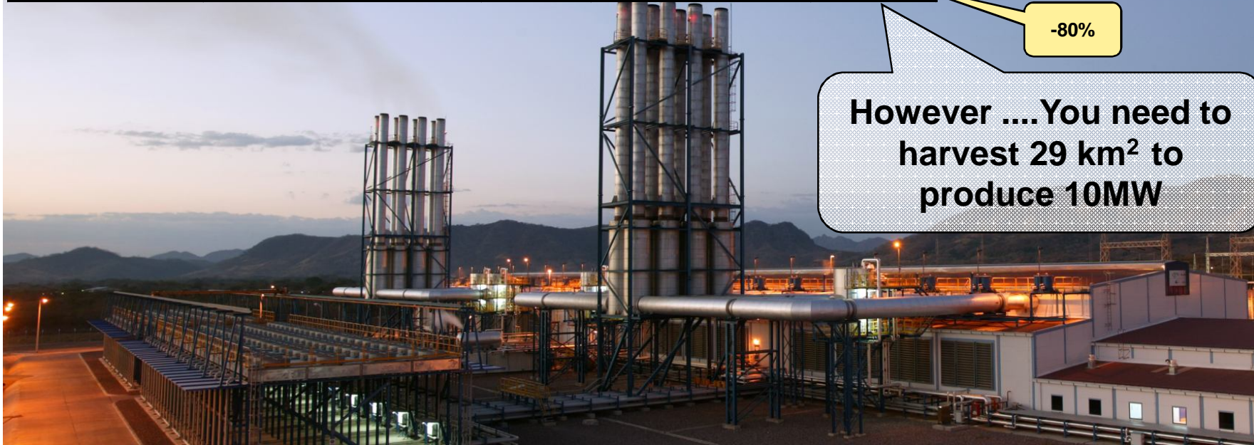
Lufussa "Pavana III" plant (Honduras): the plant accommodates 16 Wärtsilä 18V46 engines in two separate engine halls joined together by the control room.
